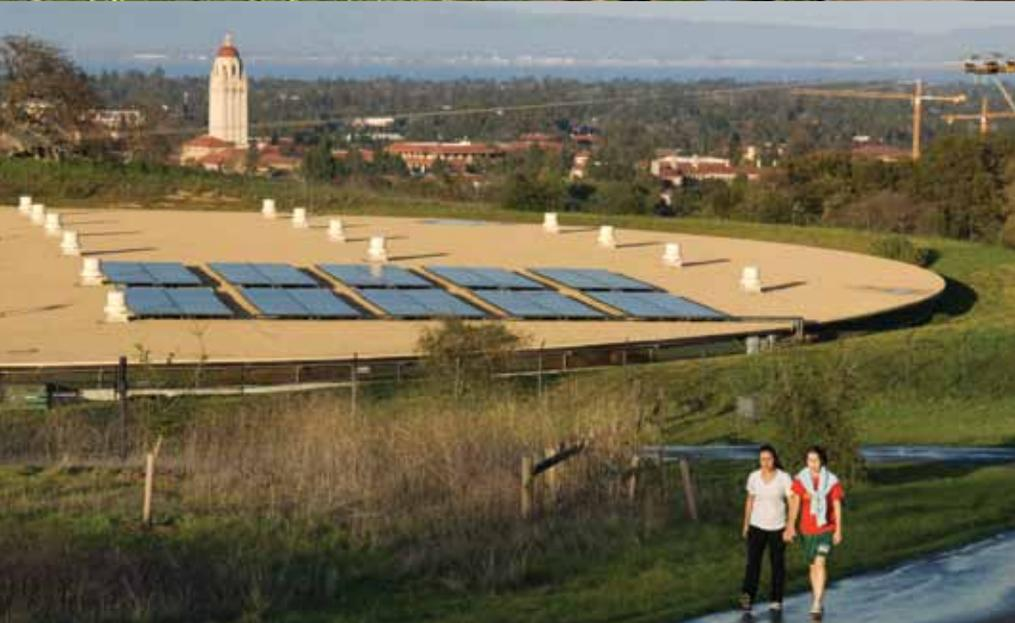
*LEFT: Hikers on their way to the Dish in the Stanford Foothills pass by photovoltaic panels that are part of ongoing sustainability efforts. The array comprises more than 200 photovoltaic modules, capable of producing 51,000 kWh each year and eliminating an estimated 61,000 pounds of carbon dioxide.*
